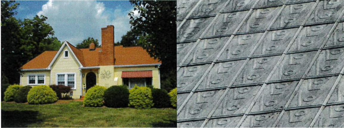
Period Cottage at 611 N. Oakland (left) and locally made metal shingles on the roof of the house at 308 N. Holland (right)
