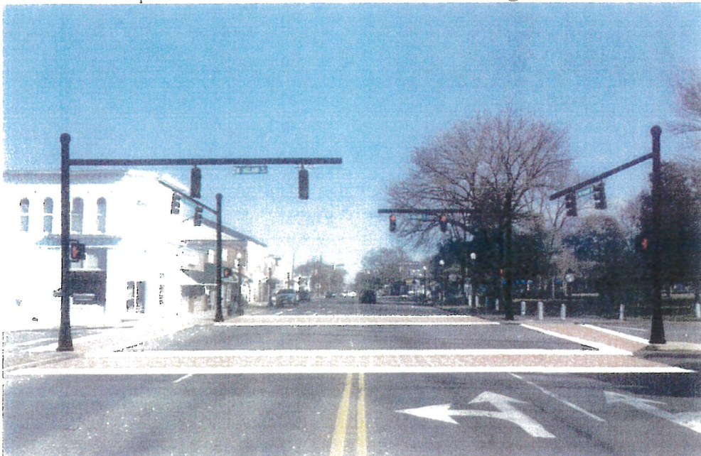
Illustration showing new signal poles and mast arms, and brick-pattern crosswalks. Note: black signal housings are used.
