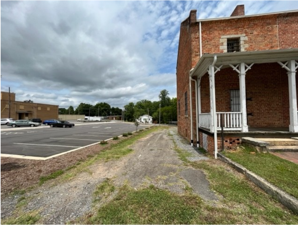
View of adjoining property facing north
