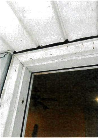
Open air gap above front door
