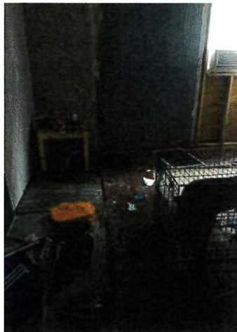
unfinisher floors & walls
