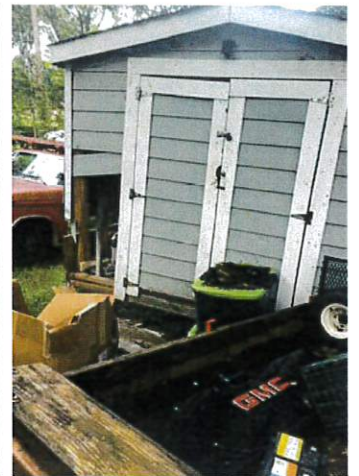
missing string- accessory structure
