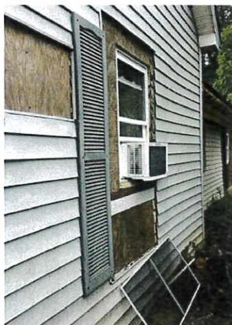
Plywood covering old window openings (re-sized)
