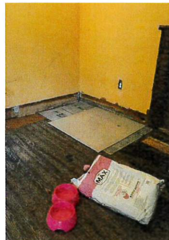
unfinished floor material
